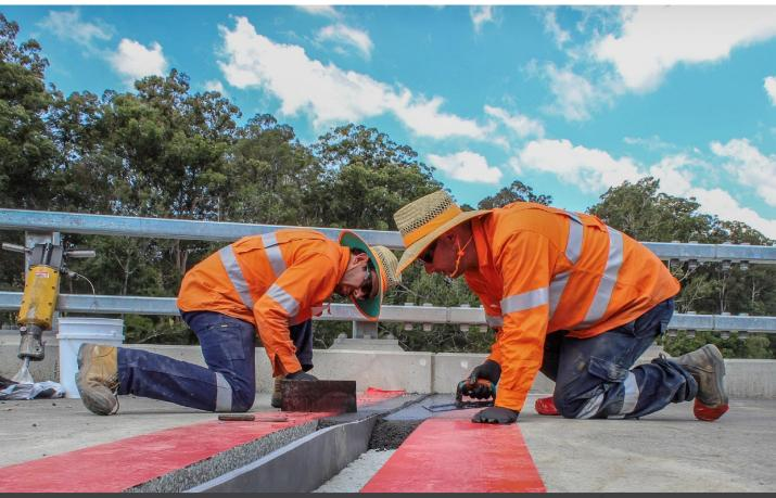
Bridge Expansion Joints enable movement and provide water tightness to bridge structures – correctly installed Expansion Joints are vital to maintain the longevity of a bridge's structural adequacy.
