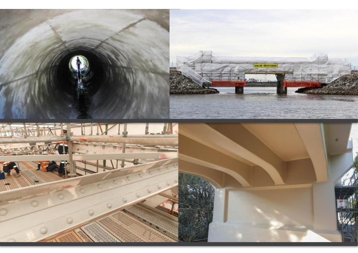
Protective coatings can not only repair **construction defects**, but they can also provide vital protection to the structure and assist in its ongoing **serviceability** and durability.
